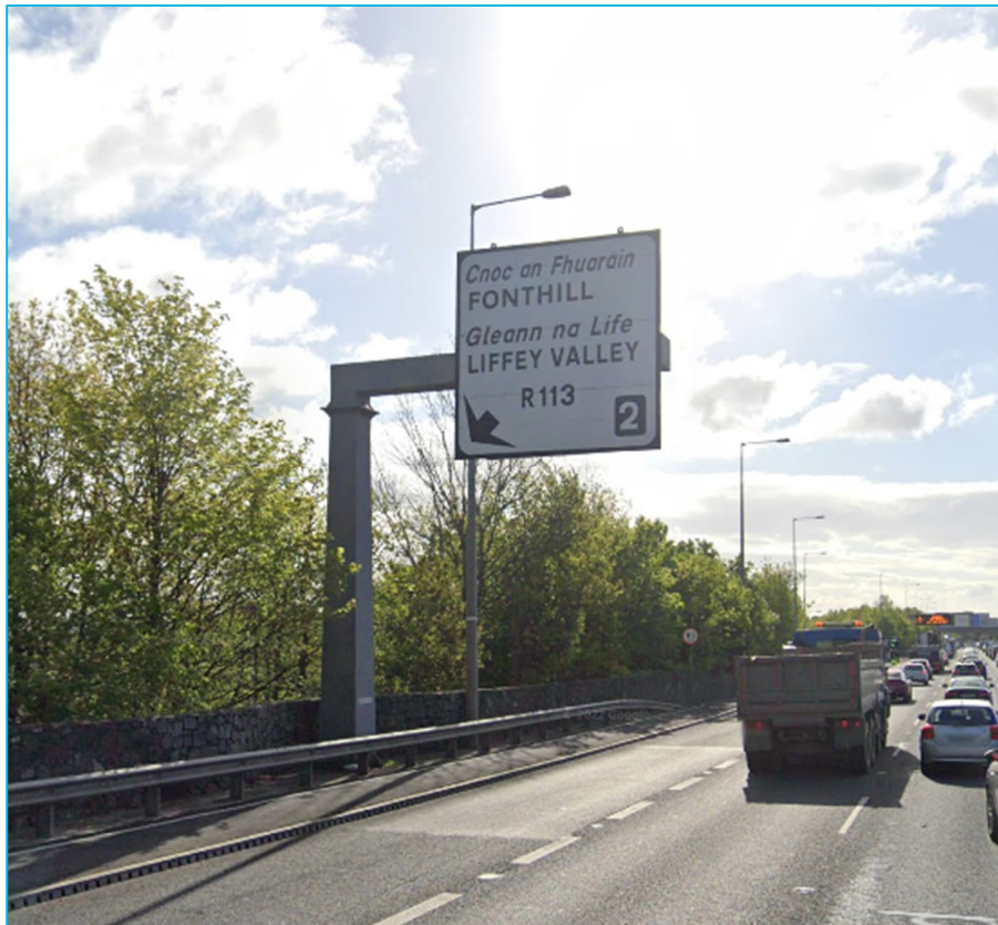
Figure 8-1 GY01 Cantilever Gantry
